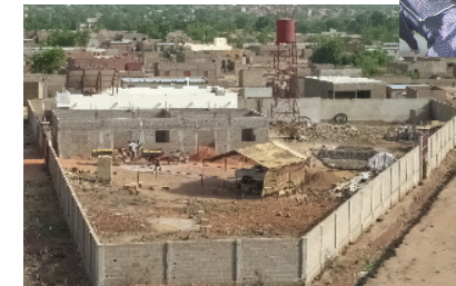
BUILDING A BASE FOR 200 CHILDREN AND WORKERS
